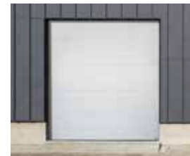
REPAIRED DOOR WITH AMARR 2747 REPLACEMENT SECTION
